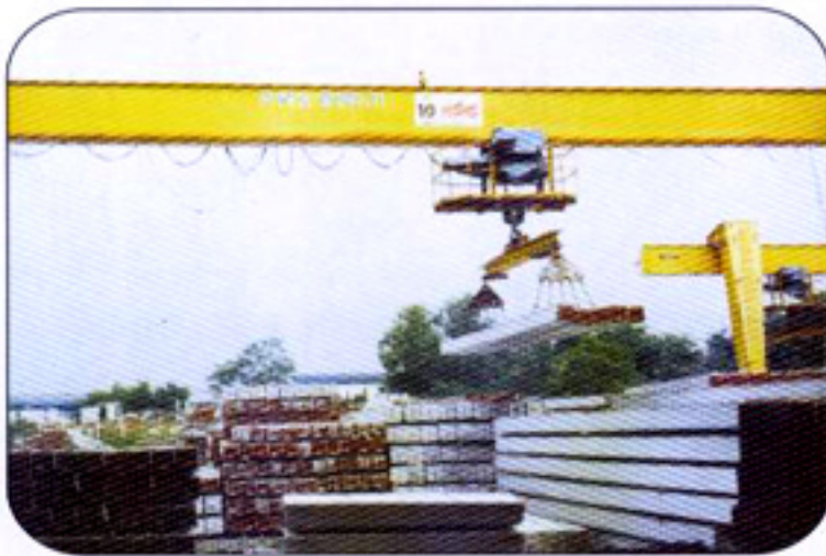
Handling at yard
