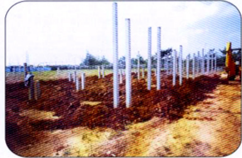
Piling work in progress
