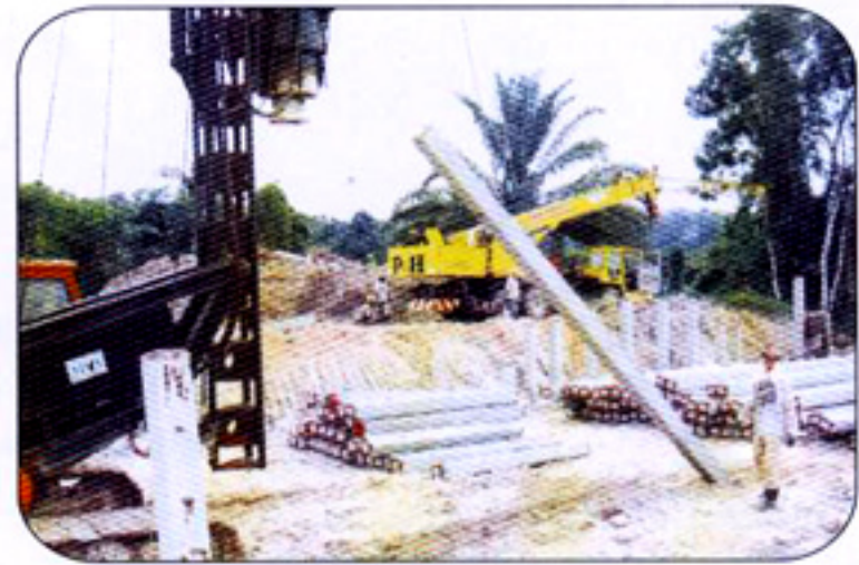
Pitching at site
